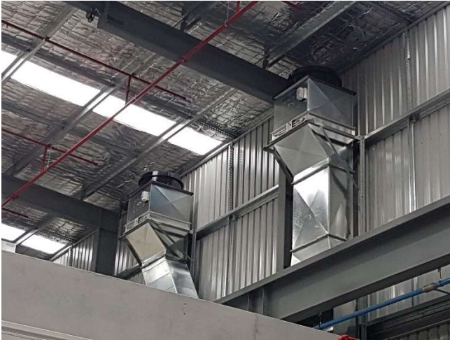
Images Above & Below: Installation of inflow supply and exhaust air ducting.
