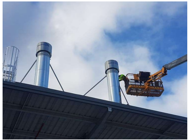
Images Above & Below: Installation of inflow supply and exhaust air ducting.
